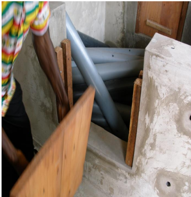
View of Door to final chamber (for removal of finished compost)
