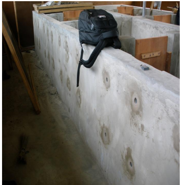
View of addition of aeration holes (fitted with PVC piping)
