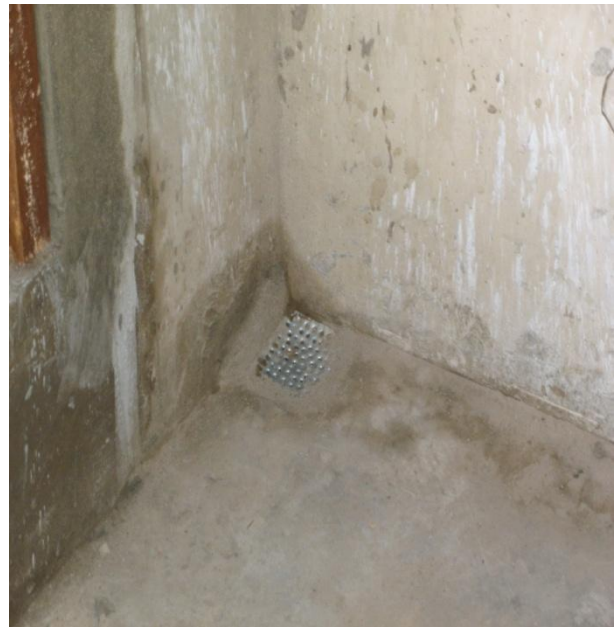
View of drain in chamber (for leachate drainage).
