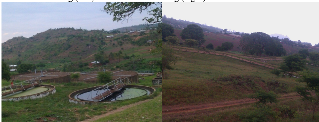
Figure 10. A Functioning (left) and Non-Functioning (right) Wastewater Treatment Plant
