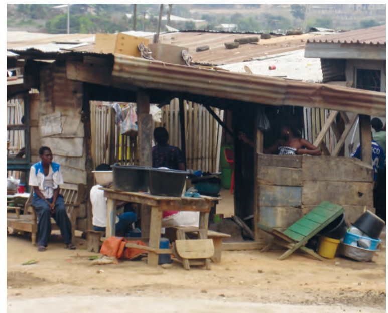
A common structure in one of Accra's under-resourced communities.
