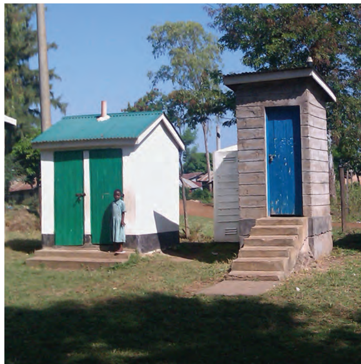
Latrines such as these can be considered improved sanitation sources with proper ventilation.
